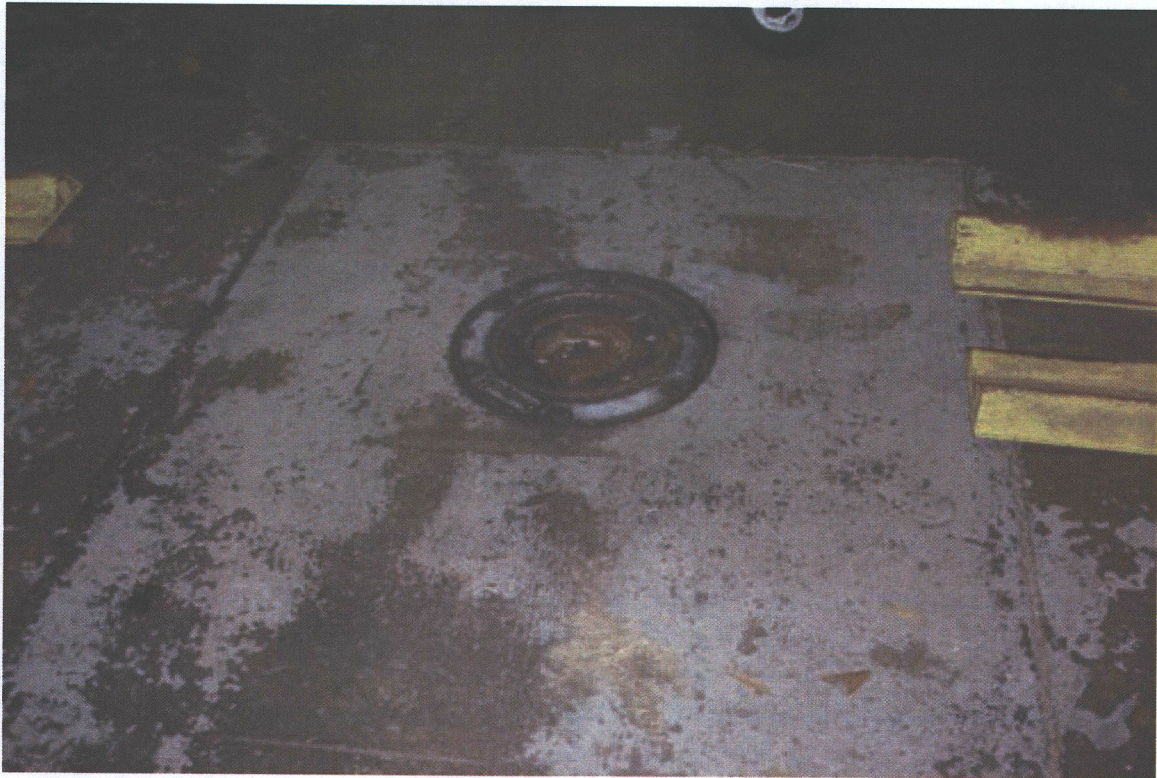
3. View of the in-ground lift located inside the service garage structure.
